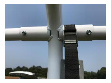
The story is not over..... After the first windstorm hit last weekend, everything went well except the structure was coming apart at the joints. So, **JR** and **Boh** drilled holes and added self tapping screws to firm up the structure. Okay, wind... your move.....
